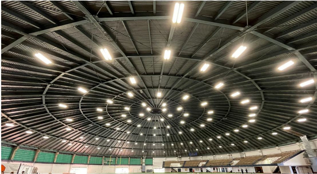
Figure 8: New LED fixtures installed in the Lally Arena.
